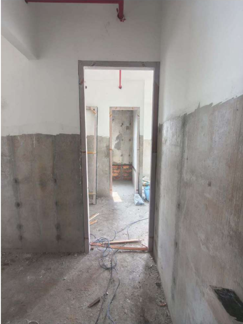
TOWER-1 - DOOR-FRAME-FIXING-WORK-IN-PROGRESS
